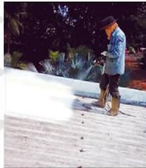
PUF Spray on Asbestos Roof sheet
