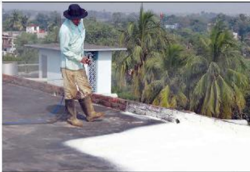
PUF Spray on Roof top of Cold storage
